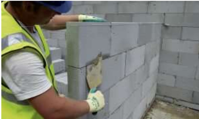
Figure 19 Thin Joint Masonry Technique
