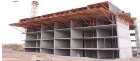
Figure 15 Tunnel Formwork System
