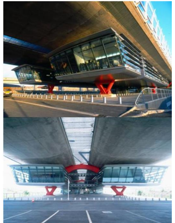
Figure view of :The A14 highway elevated road and control centre
