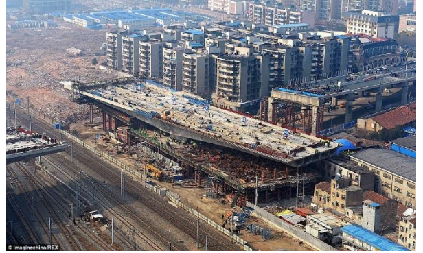
Figure-swing bridge rotation 0 degree
