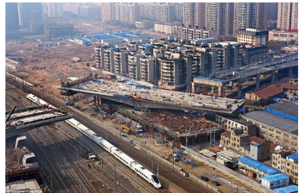
Figure-swing bridge rotation 45 degree
