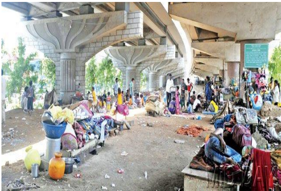
figure- uneven parkings/dhobi-ghat under flyover
