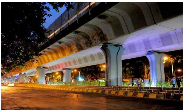
Figure-matunga flyover ,Mumbai
