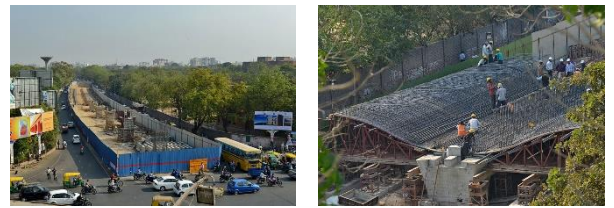
figure –AMC flyover at IIM junction flyover ahmedabad durning construction
