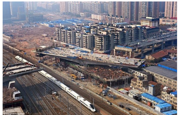
Figure-swing bridge rotation 30 degree
