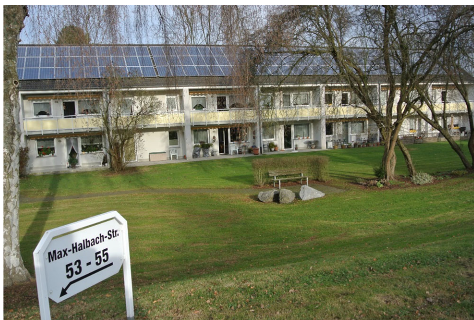
Figure 1: Max-Halbachstraße 53–55: one of the few remaining assets of FdR in Mülheim an der Ruhr (source: photo taken by Annia Martinez) [Colour figure can be viewed at wileyonlinelibrary.com ]
