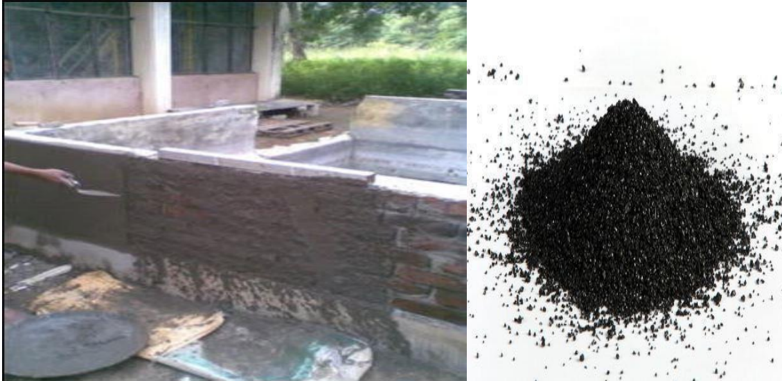
Figure 5. Plastering with Copper Slag and Raw copper slag material.
