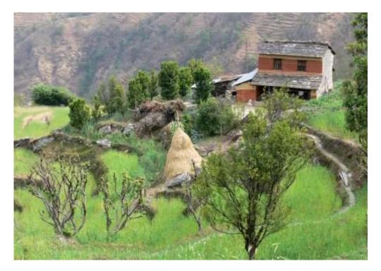
The traditional Nepali house design consists of thick stone walls, a thatched roof made of either hay, stone, or tin, and a paste of manure and clay (kamero) for the painting. They also have wooden pillars.
