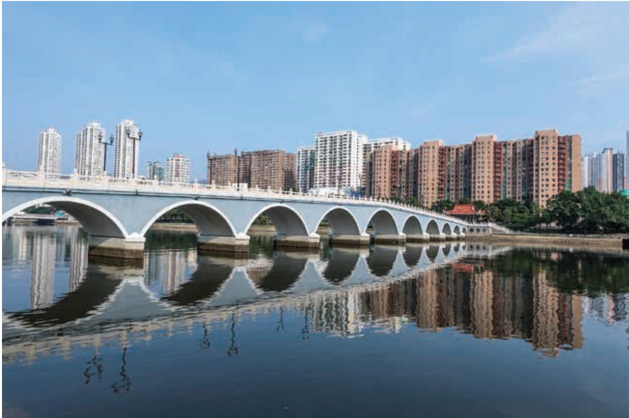
Sha Tin Urban Development (Housing) Project in Hong Kong, China. The project is ADB's first in the urban development (housing) sector (photo by ADB).
