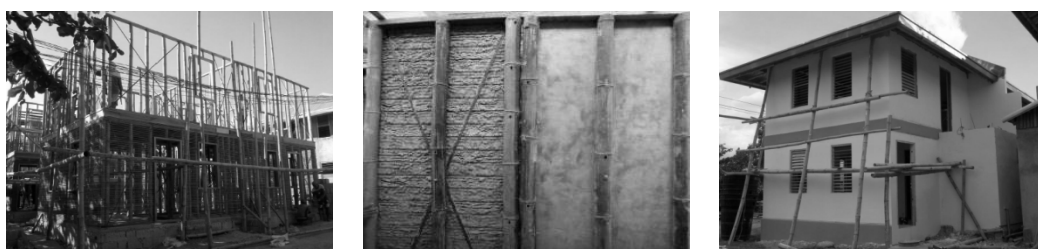
Figure 10. Modern bamboo-based housing built in Iloilo, Region IV in 2015 by [46,49].
