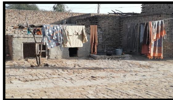
Improper Internal Layouts
