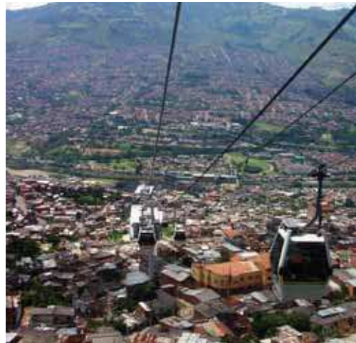
Metrocable Line K with the Medellín river in the background © Julio D. Dávila 2010
