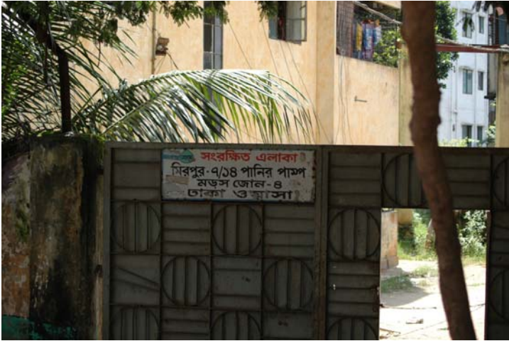
Picture 9.1.2b: Water pump station run by DWASA located next to Jhilpar; (Source: Author, 2008)
