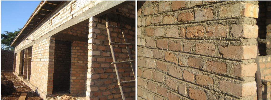
Figure 10: Excessive use of mortar due to uneven sizes/shapes of bricks.
