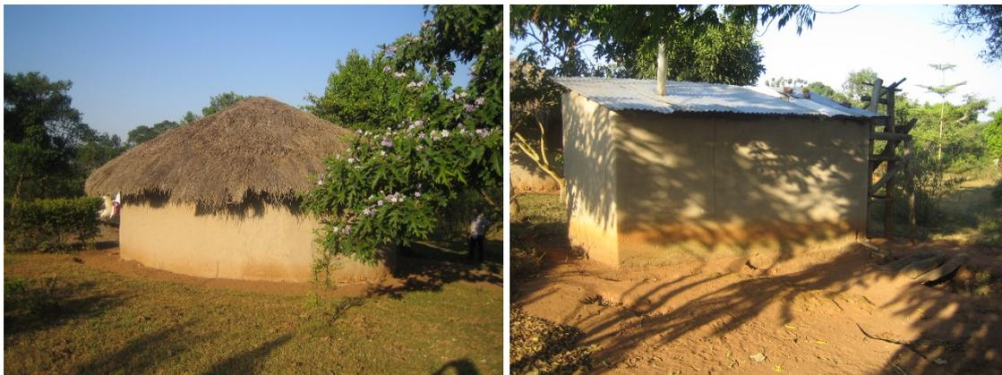
Figure 6: Thatched roof (left) and Iron Sheets roof construction (right).
