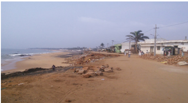
Image 3: Damaged Road during Cyclone Hud-Hud near Bhimunipatnam
