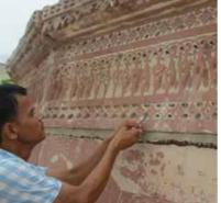
(Above) Dismantling of the cement plaster from the drum of the dome; Restoration work of the finial made in red sandstone; Careful removal of multiple layers of the paints from the ornamentation work of the dome in red sandstone.
