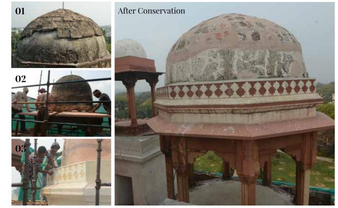
(Left column images) As with other portions of the structure, the four corner canopies were covered with cement layers, these have been renewed, the cracks repaired with traditional lime mortar; (Right) After conservation view of the canopy after removal of cement and restoring the fallen chajjas/eaves.
