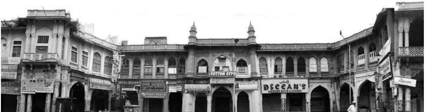
A view of the Pathergatti Arcade façade with commercial signage, 2006
