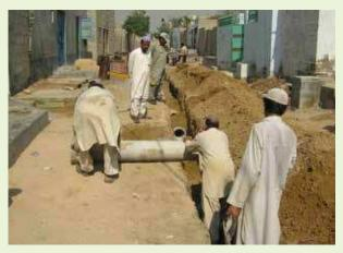
Construction of a self-help lane sewer in Gulshan-e-Zia. Street scene: during laying of sewerage pipe on self-help (background: OPP-RTI technical advisor supervises). Photo: Orangi Pilot Project.
