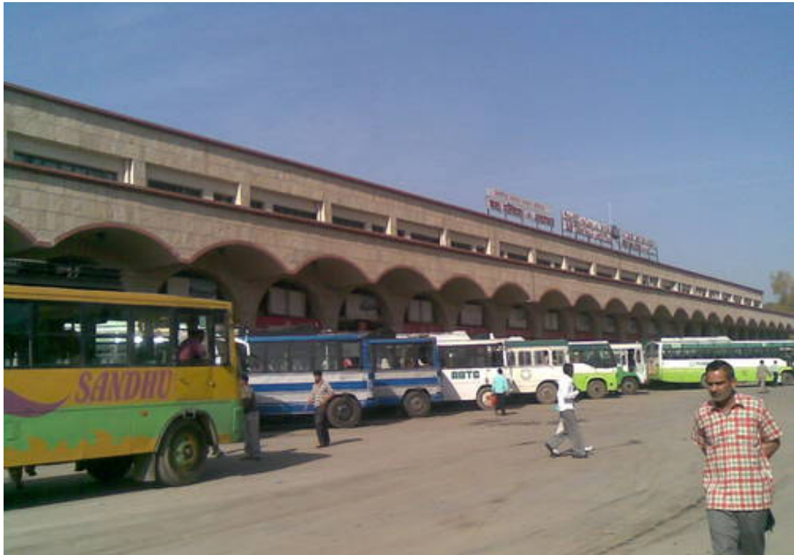
Photograph 3.6- New and Improved Bus Stand Developed under PPP Model
