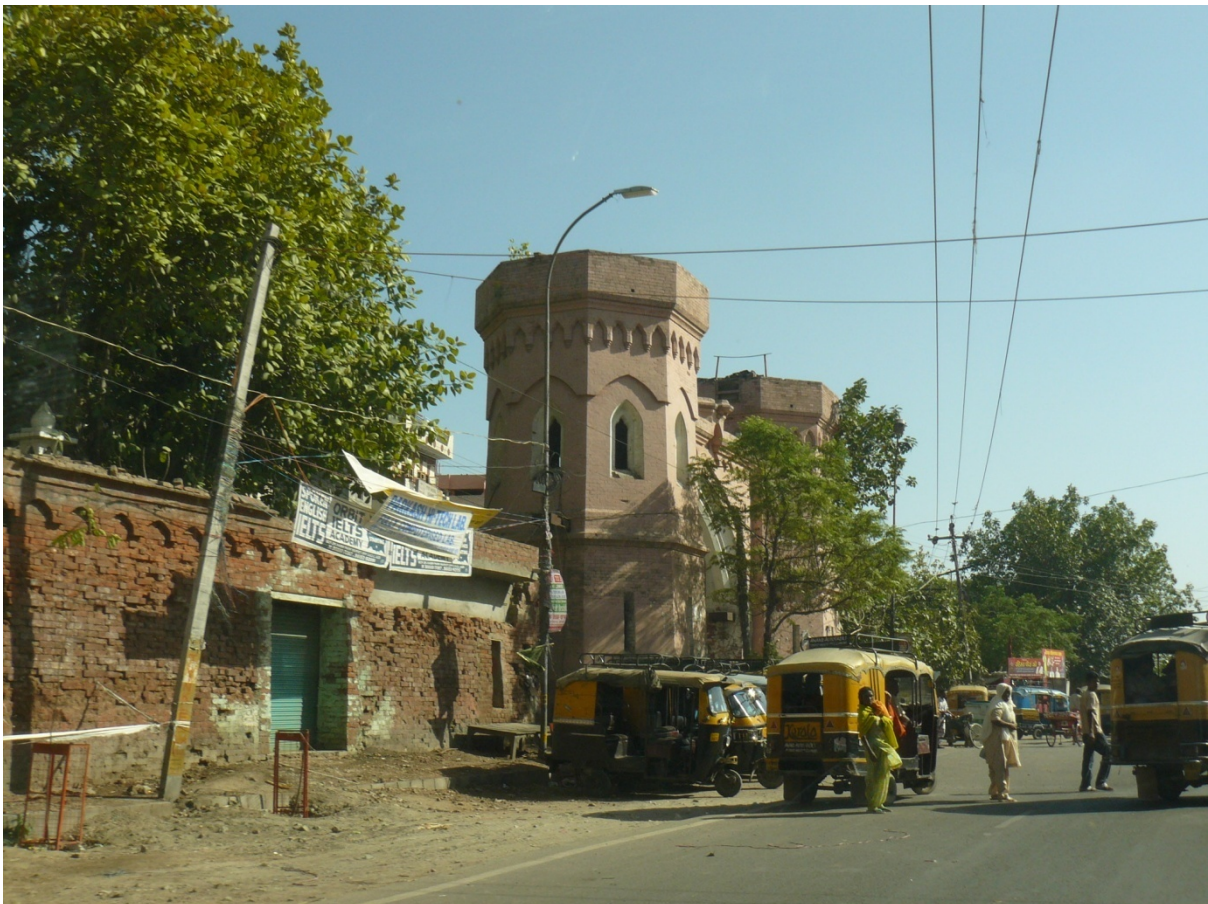
Photograph 3.2-Gate and Wall around walled city- depilated condition (Amritsar)
