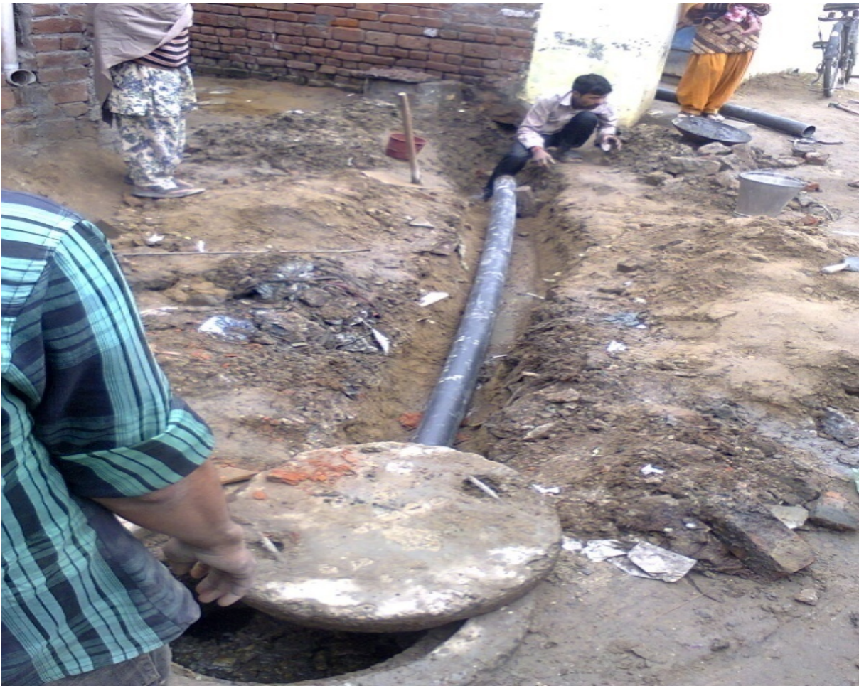
Photograph 8.2_ Laying Sewer in Unplanned Areas in Amritsar (Kot Khalsa Area)
