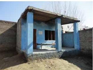
Above is a picture of Basheer Khan Shah Rawan's house. It was constructed of cement blocks and by recommendation of NRSP GM Agha Javad steel rods were inserted in the corners of the room to meet safety standards and to strengthen overall foundation. The plaque above was installed outside each house constructed as a result of the Express Helpline Trust grant.
