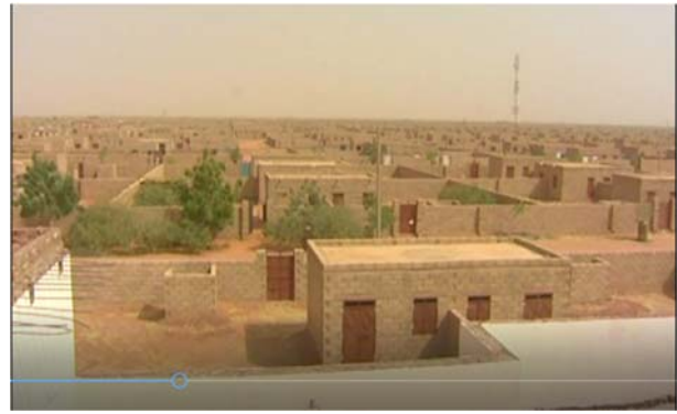
Figure (9): Aerial View of the core-unit of
