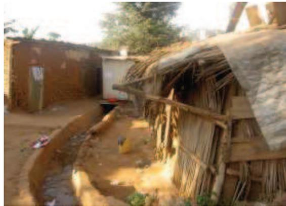
**Fig. 2:** Papyrus used for constructing temporary structures
