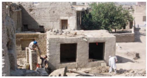
Figure 32: Load-bearing masonry construction is common in most Central and Western Asian countries, and is typically well suited to the climate and local resource availability. Photo © UN-HABITAT
