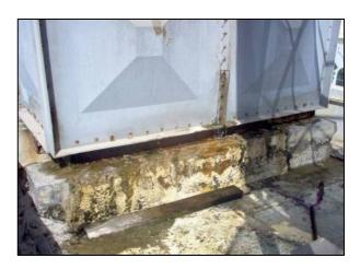
Figure 6. Damaged Water Tanks
