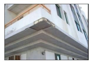
Figure 8. Falling of External Marble Cladding
