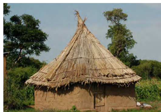
Rectangular chikka house with a papyrus roof in Oromia. Papyrus is less durable but easier to build with as it grows faster than grass. © Lorenzo Fontana
