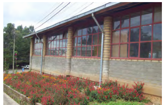
School built with CEB (Compressed Earth Blocks) in Addis Ababa. © O. Moles- CRAterre
