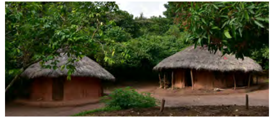
Aari houses built on a mound with a round verandah protecting the walls from the rain. (Dehub Omo Zone in SNNPR). CC- Richard Mortel
