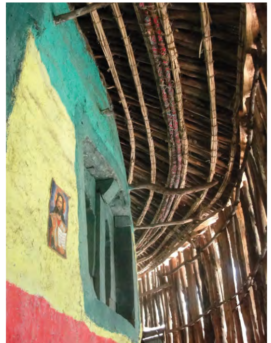
Church in Bura (Amhara) with an inner block built with chikka protected by a roofing with a very large overhang that creates a verandah surrounding the entire building. An eucalyptus screen helps protect the chikka mortar and the foundations of the inner block from black cotton soils cracking. © L. Davis
