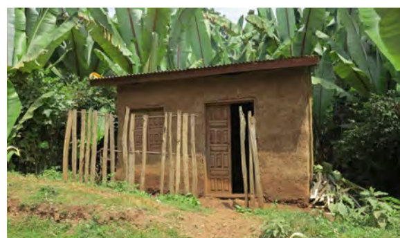
Chikka house in Gedeo Zone (SNNPR). © ShelterBox
