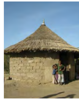
Adobe round house in the Ethiopian Rift Valley (20 years since construction). © Petersson & Strom
