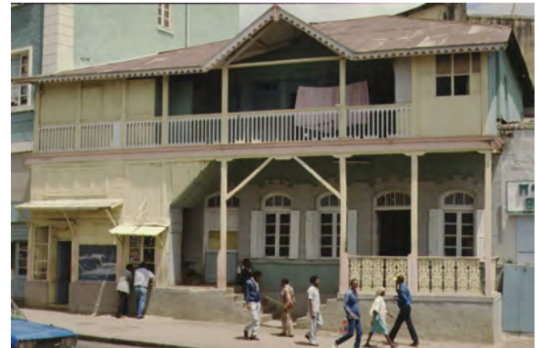
Addis Ababa style building with verandah. ©T. Joffroy-CRATERRE
