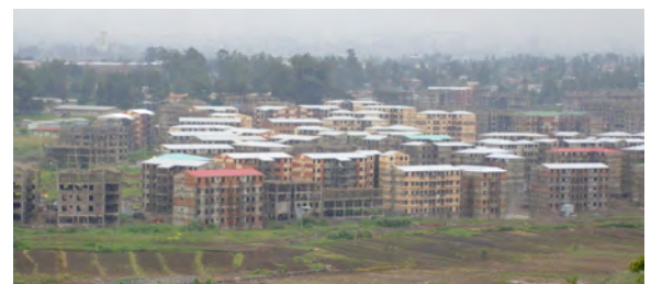
Condominiums under construction Addis Ababa. CC- Maguns Franklin
