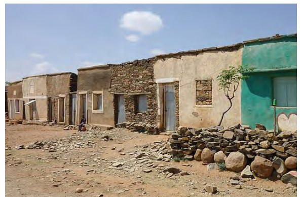
Houses with stone masonry walls in Tigray. CC- Bernard Gagnon
