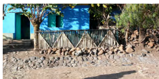
Surface drainage system to prevent from erosion and flooding near Bahir Dar, Amhara. © O. Moles
