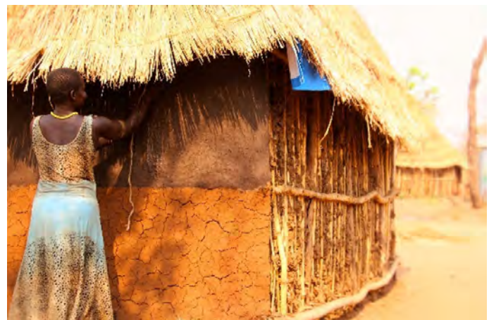
Active participation of beneficiaries through mud plastering and thatching. © Muse Mohammed - IOM
