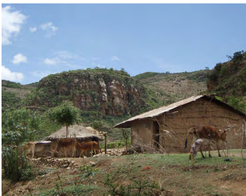
Square chikka house with CGI sheet roof and round chikka house with thatch roof in rural Dire Dawa. CC- Petr Kosina
