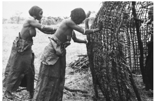
Construction of a Borana «bird's nest» house. CC- National Museum of World Cultures
