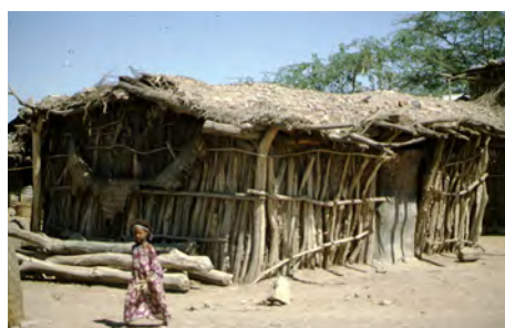
Permanent constructions with wooden structure and earthen roof in Afar region. ©T. Joffroy- CRAterre
