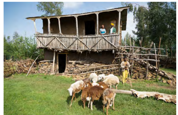
Two story house with stone plinth, chikka walls and balcony in Gogbob village, Amhara region. CC- Kelley Lynch USAID
