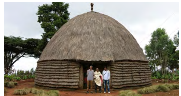
Welayta people house built with a bamboo structure and a vegetal covering. © Todd McGowan
