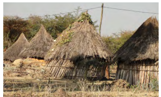
Stability problems due to black cotton soil expansion and contraction near lake Tana (Amhara). © L. Davis
