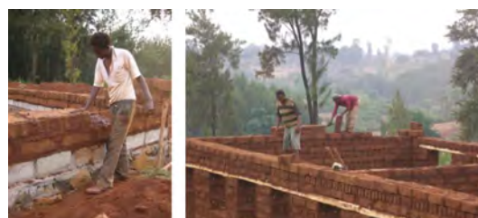
Adobe construction in Aira (Oromia). © Petersson & Ström
