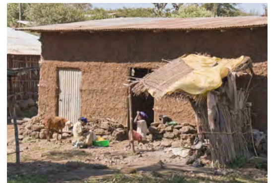
Stone masonry wall built to protect the lower part of the chikka walls in Bahir Dar. (Amhara). CC- A. Davey
