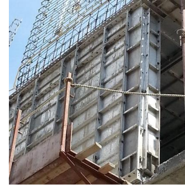
Fig. Aluminum Formwork used in wall construction
