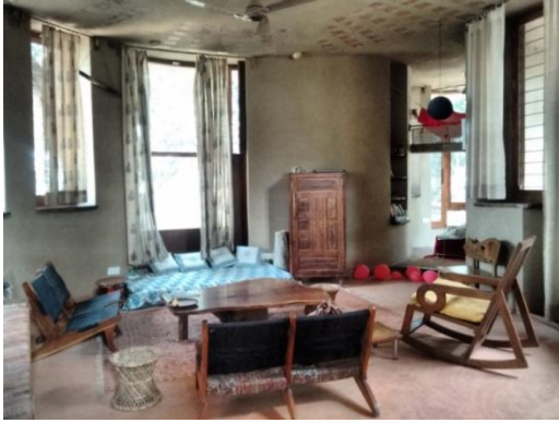
Figure 34 Living space with terracotta filler slab
