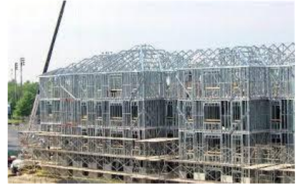
Fig. Light Gauge Steel Construction
