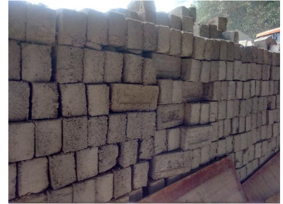
Fig. C&DW Blocks used in wall construction
