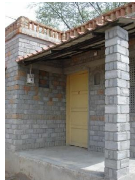
Figure 46 The entrance porch of a house (DevelopmentAlternatives 2010)
