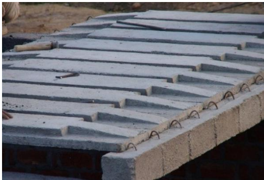
Figure 47 Use of precast Ferrocement elements for first floor slab (DevelopmentAlternatives 2010)
