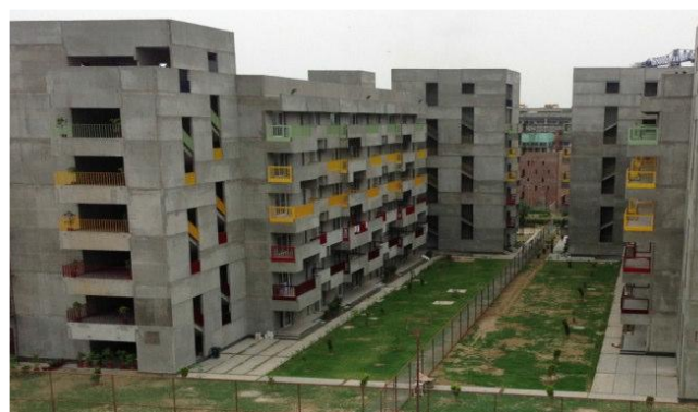
Figure 27 Pre-cast panel construction in O.P Jindal University, Sonipat
