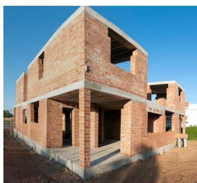
Figure 10 Load bearing brick work construction with RCC slab
