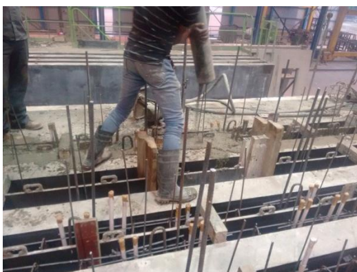
Figure 29 Concrete pouring in pre-cast mould for wall panels
