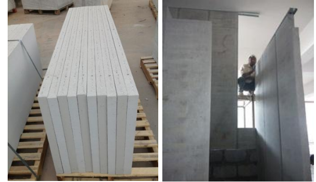
Fig. cement fiber board ; Interior dry wall construction
