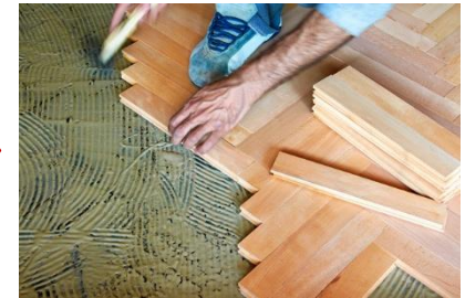
Fig. Parquet flooring Installation (from recycled wood)
