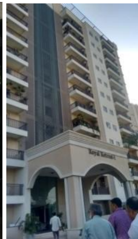
Figure 14 High rise housing by Omaxe builders
