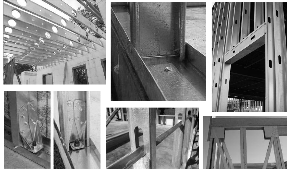
Fig. Light Gauge Steel Construction.
