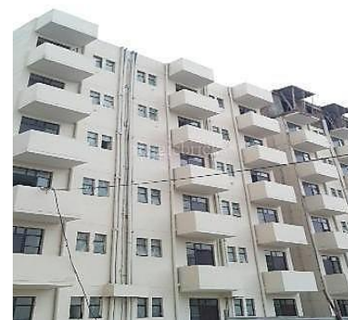
Figure 16 EWS Housing by ASCC for PHDB
