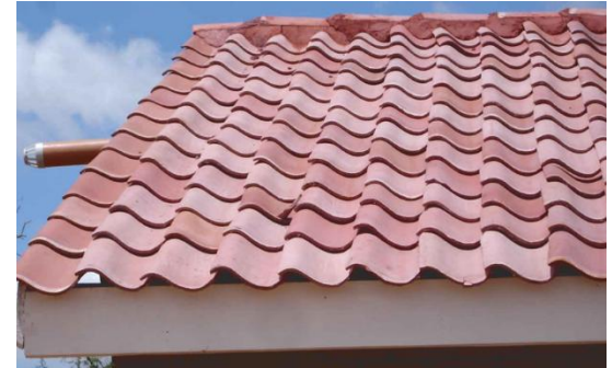
Fig. MCR Tiles used in roofing construction
