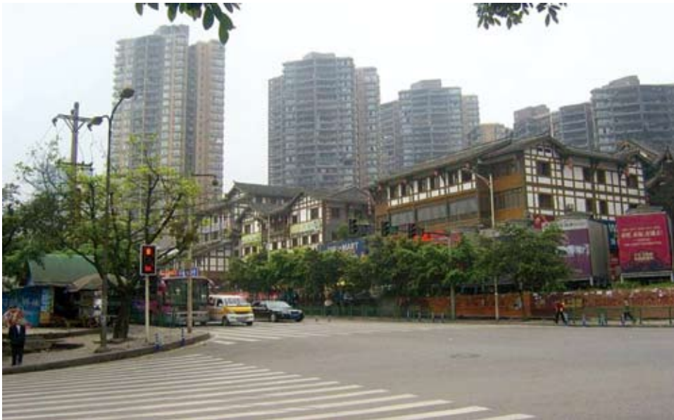
Typical Post 1994 High-Rise Housing in China (Chongqing) Source: The Authors
