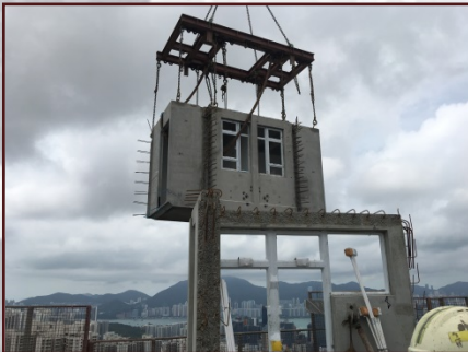
Volumetric precast bathroom & kitchen
