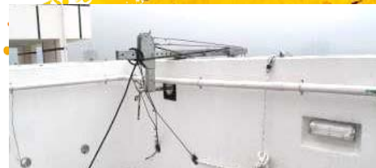
Strengthened Parapets to fix gondola
