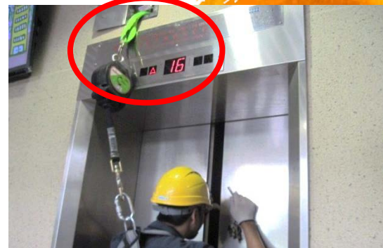
Permanent anchorage to access lift pit
