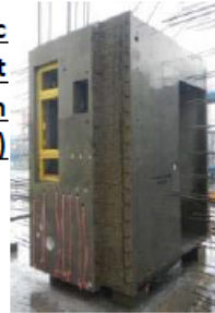
Volumetric Precast Bathroom (VPB)
