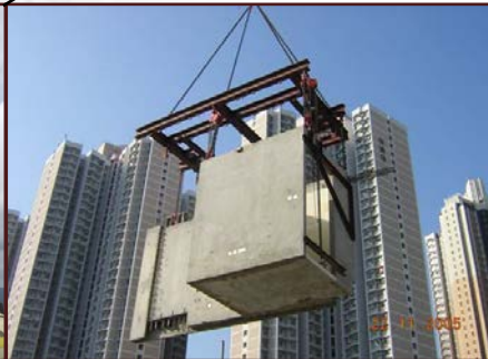
Volumetric precast bathroom & kitchen
