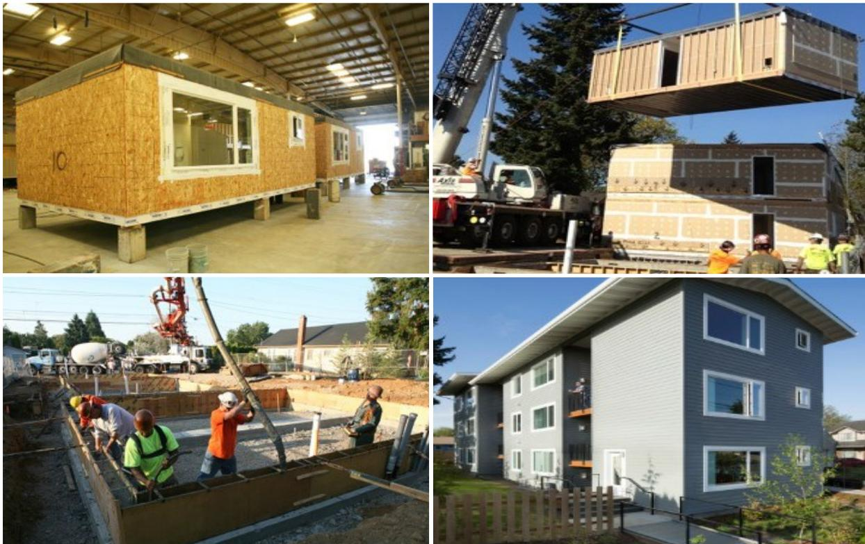
Modular housing can be assembled in the factory while the site preparation work is being completed. Once the modular units are delivered to the site, the buildings go up quickly.
