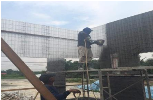
Figure 9: Concrete Spraying Process on the EPS Panels
