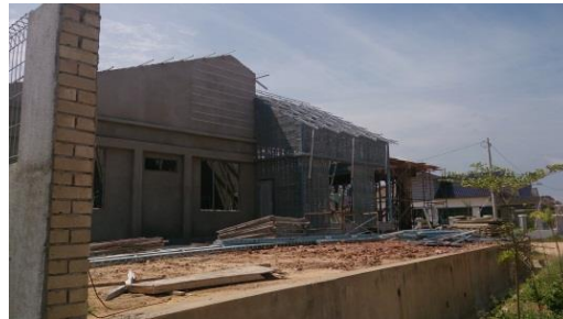
Figure 6: House Built Using IBS Steel Framing System
