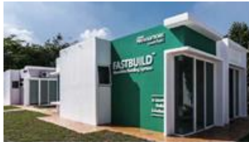
Figure 4: House built using On-Site Monolithic Building System
