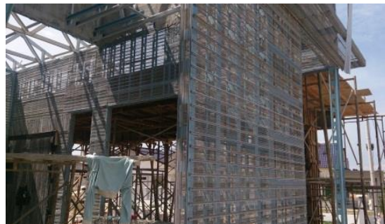
Figure 7: The Erection of the Lightweight Steel Framings into a House
