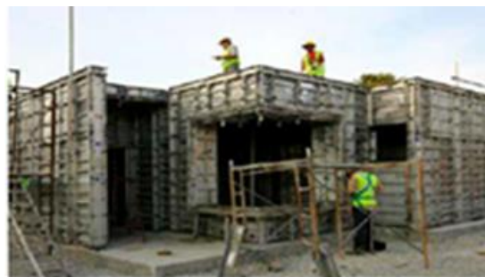
Figure 5: Formwork Installation On-Site
