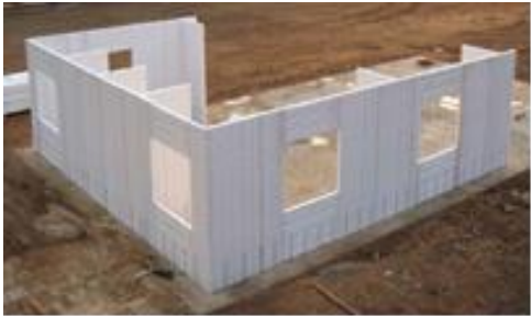
Figure 8: House constructed using IBS Innovative System (EPS)
