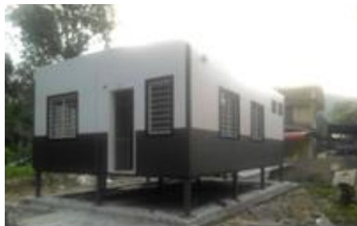
Figure 1: Modular Prefabricated House
