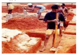
Fig 2: rammed earth foundation
