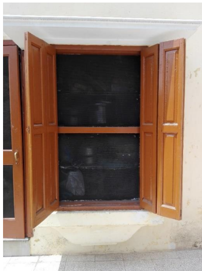
Figure 12: Cooling cabinet used before refrigerators, built 1937. Case-study 3
