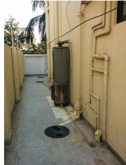
Figure 15: Outdoor peripheral spaces in contemporary house. Case-study 5
