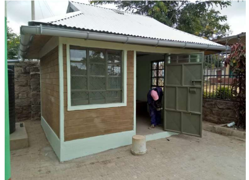
SSB house featuring rainwater harvesting
