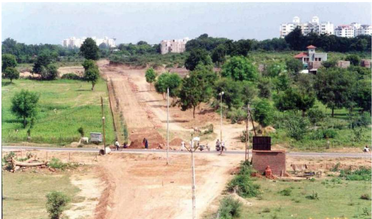
Figure 6. Construction of Roads After Approval of Draft TPS
